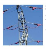
BCIC covers for Dead End connection points and Suspension Clamps protect energised lines from perching, landing and nesting birds.
